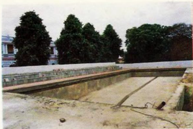
The Swimming Pool (Under construction) 1996
