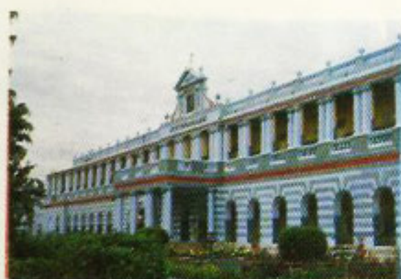
Main Block (View from Right Corner)
