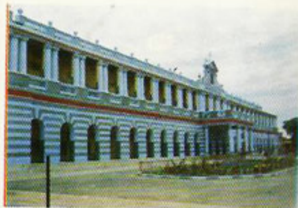
Main Block (View from Left Corner)
